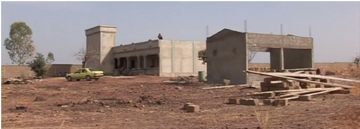
Progress of the Zorokoro Children's Complex as of December 2014
